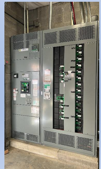
Switchgear replacement at LCHS
