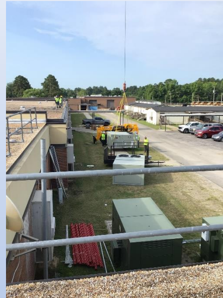
Rooftop HVAC work at LCHS
