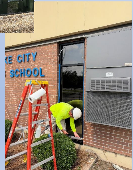
Window and film installation at LCHS
